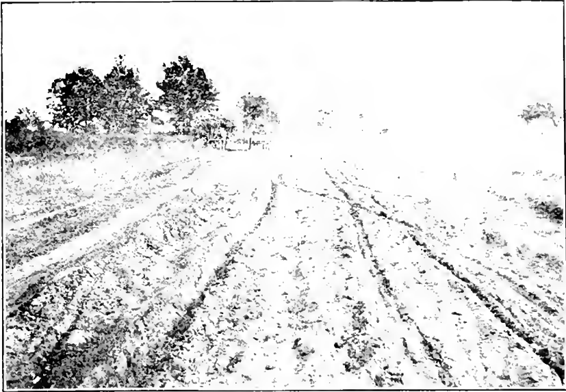
KLAYPORT AND KLANSBURG ROAD, BEFORE IMPROVEMENT.
