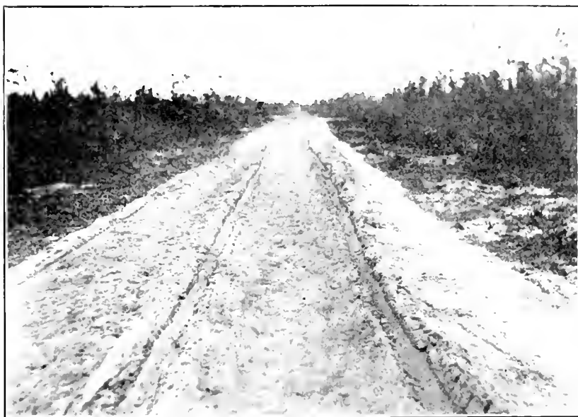
EGG HARBOR AND GREEN BANK ROAD, BEFORE IMPROVEMENT.
